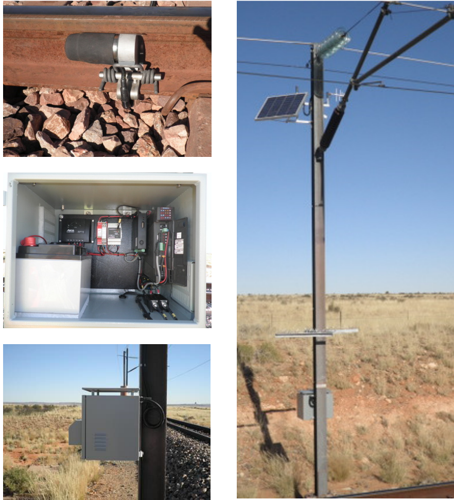
Fig. 2. Typical UBRD V4 Station Installed on ORELINE.
